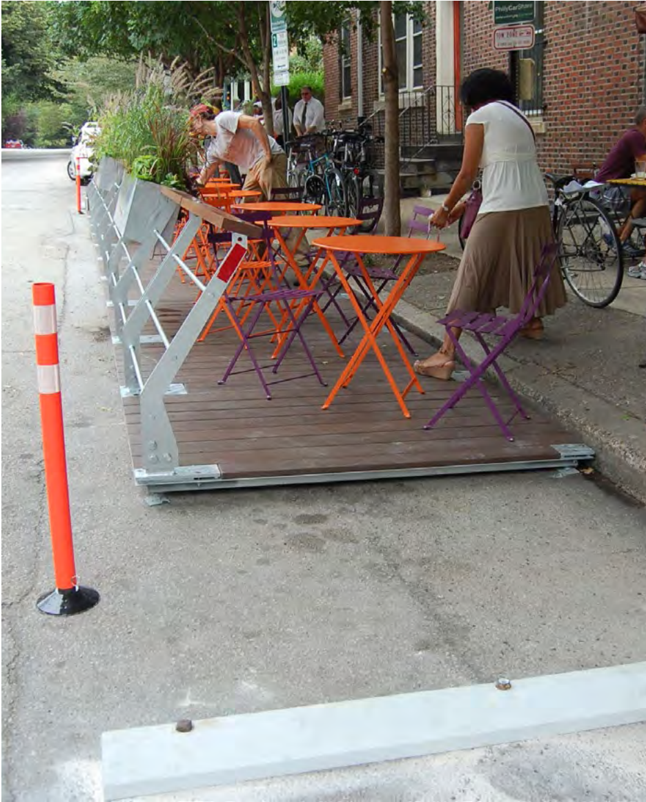
Figure 46. Wheel stop and flexible bollard, Philadelphia, PA. Credit: Philly Bicycle Coalition
