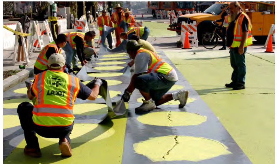
Figure 61. LADOT installation crews, Sunset Triangle Plaza, Los Angeles, CA. Credit: Margot Ocañas
