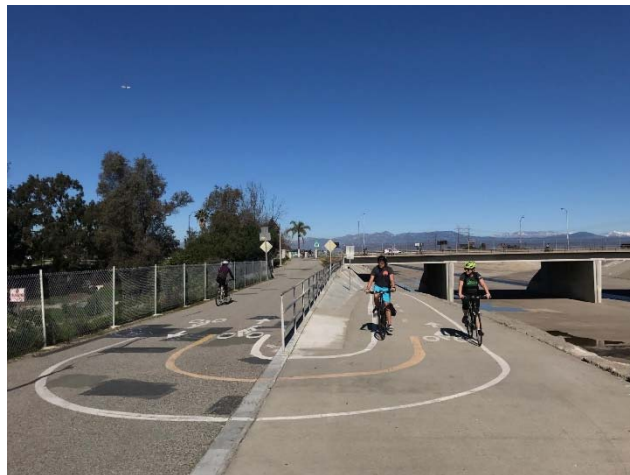
Figure 41. Narrow space for bicyclists on the Imperial Highway between two fences.
