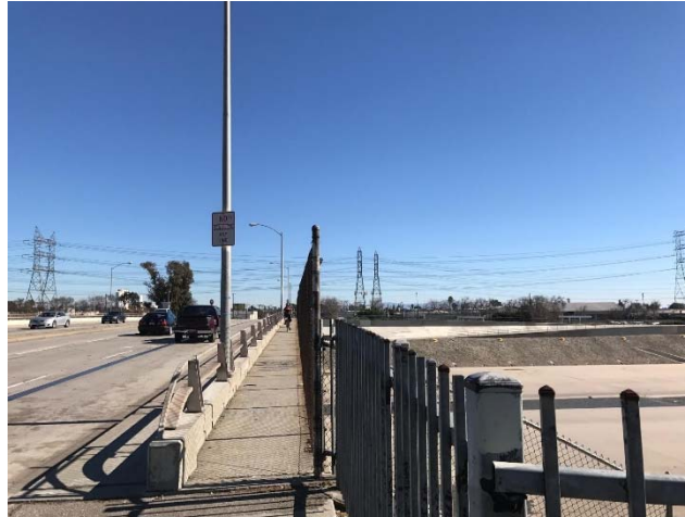
Figure 40. Picture of a 180 degree turn to access the Imperial Highway Bridge.
