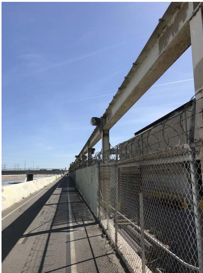
Figure 18. Commercial property separated from River Path by fence, barbed wire & lighting.
