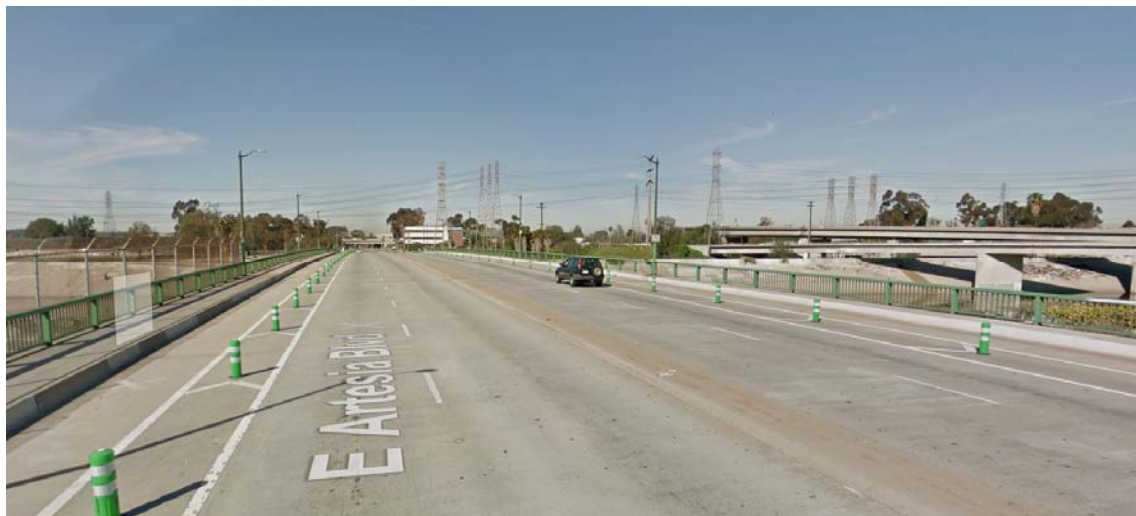
Figure 43. Above protected Bike Lanes on the Artesia Boulevard Bridge.
