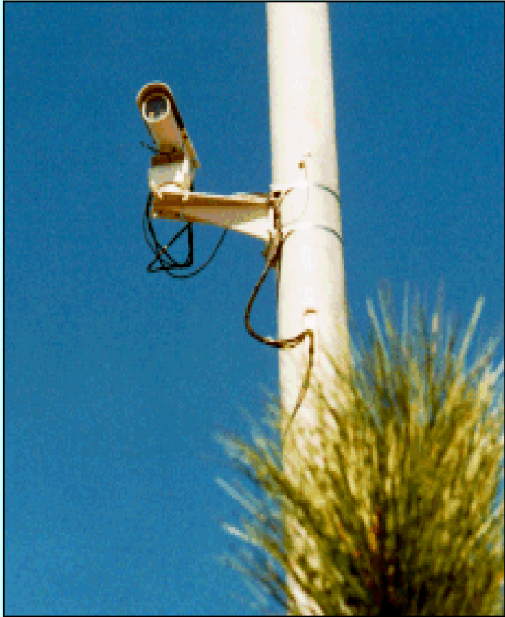
Traffic Cameras (CCTV)
